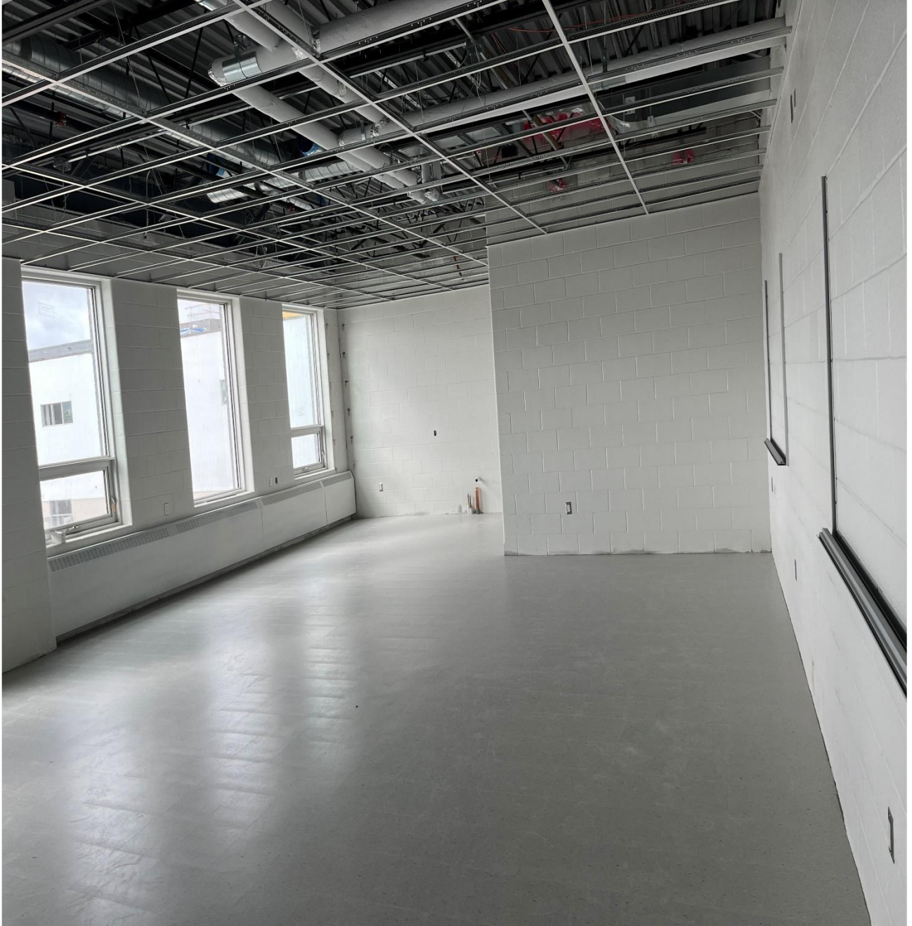
Finishing work is ongoing in classes room in par A
