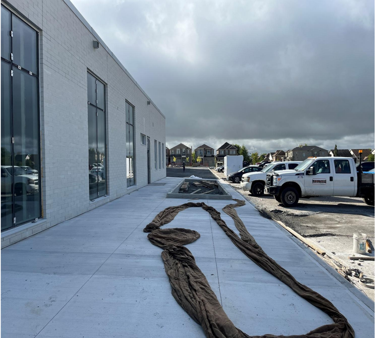
The concrete sidewalk around the elevation ongoing
