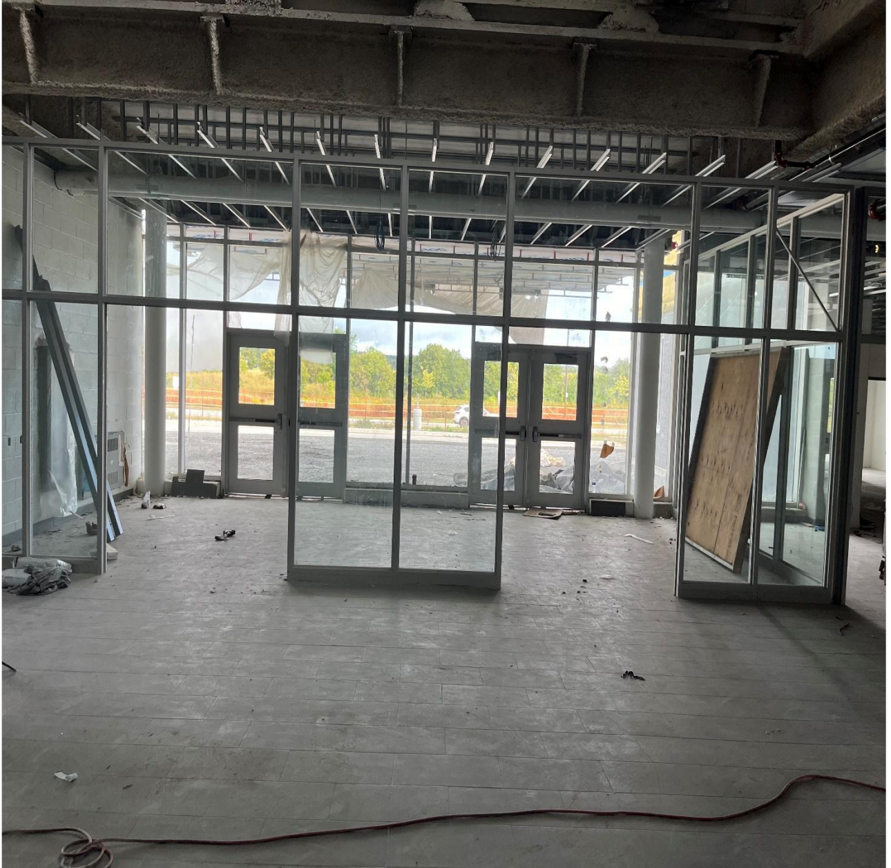
View of going work in enters aluminum doors and tiles
