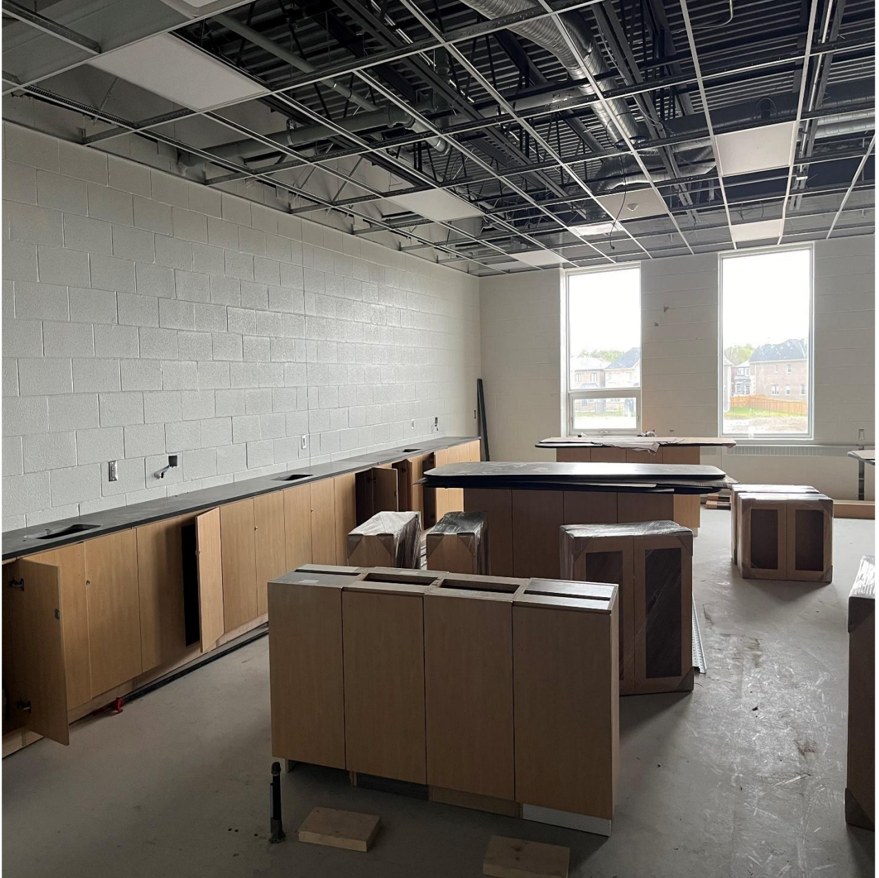
The millwork is currently in progress in the lab
