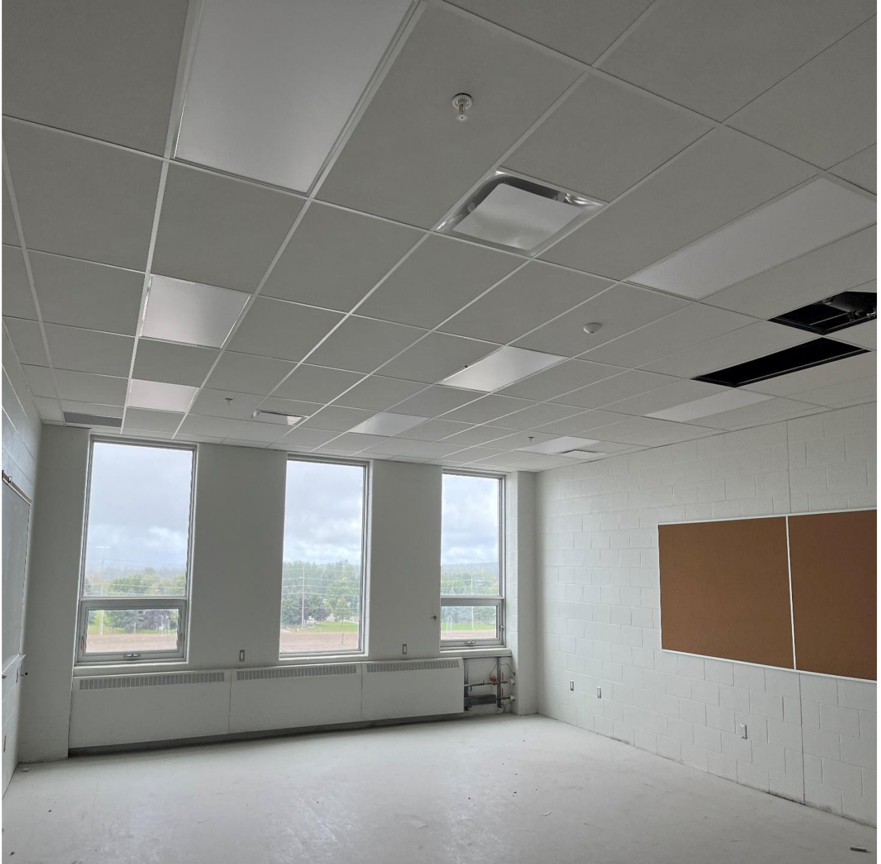
Ceiling work closing and Board work in progress
